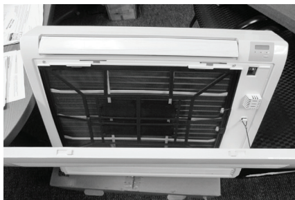
Figure 7. MFMA Typical Filter Removal
